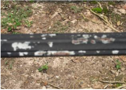
Properly prepping the rails will ensure proper adhesion.
